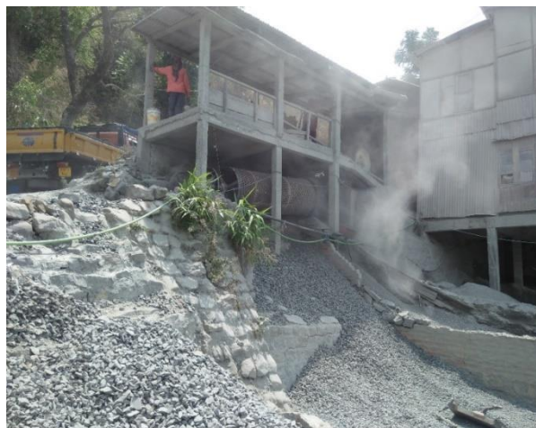
Plate 3.3.2: A crusher site
